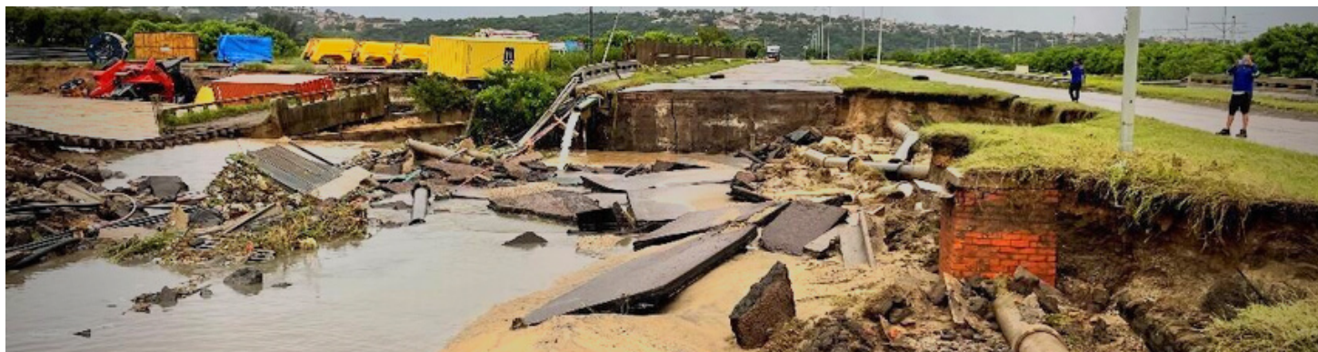
Site of the damage caused by floods in KwaZulu-Natal Province
