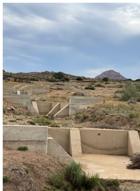
A gabion being constructed to prevent erosion
