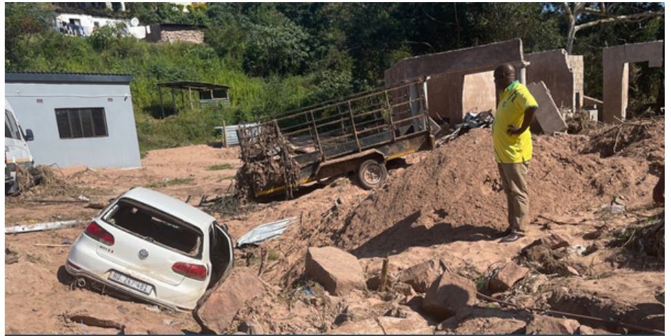
A car remains stuck in the ground two months after KZN floods damage
