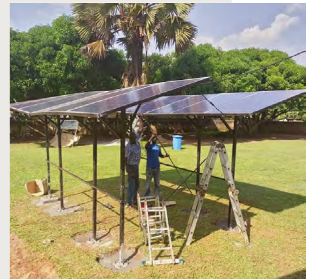
Installation of solar panels at OHCHR in Panama and in Uganda. © OHCHR
